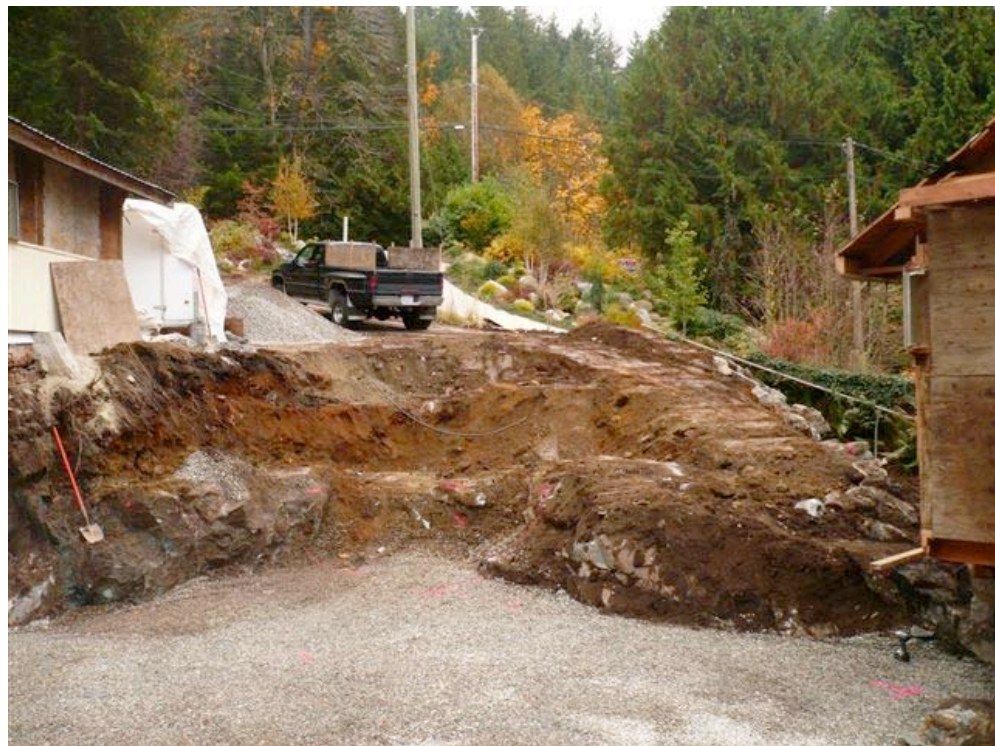
Figure 8. Photograph of landscape taken by the contractor Mark Wilson during development activities. Photograph is taken of general area prepared for house construction and displays blasted rock and indigenous soil disturbed prior to the application of this permit.
