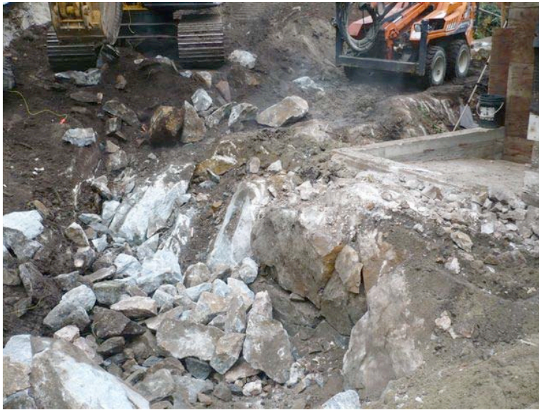
Figure 5. Photograph of landscape taken by the contractor Mark Wilson during development activities of area prepared for house construction, displaying blasted rock and indigenous soil. Photograph taken prior to the application of this permit.
